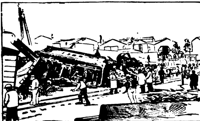
THE OVERTURNED LOCOMOTIVE AT TWENTY-SIXTH STREET.
